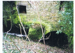
Spillway at Fulwood Mill (NB: Private Property)
