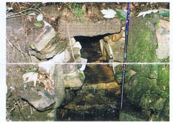
Box drain elsewhere in the valley
