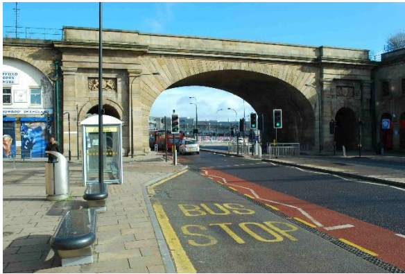
Wicker arches – the main arch
