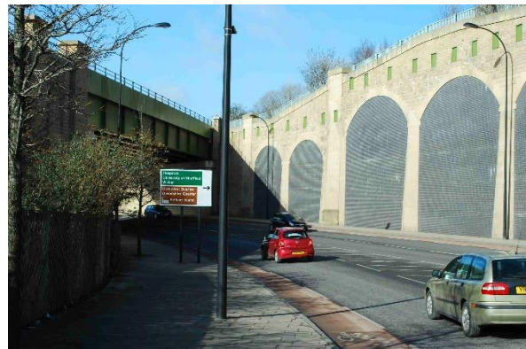
Inner relief road (Brunswick Road) - new work in Peakmoor Sandstone, recapitulating the old Wicker Arches opposite
