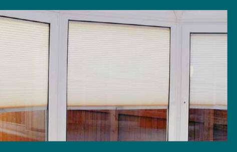
The application of Verosol pleated blind fabrics, coated with an aluminium layer on one side, reduces solar heat gain and improves the U-value, whilst regulating the light passing through. Light transfer down the blind edge is eliminated by the use of special 'L' shaped-side guides.
