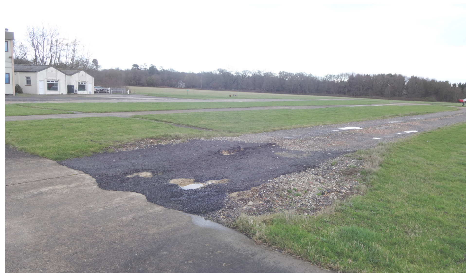
Condition of taxiways.
