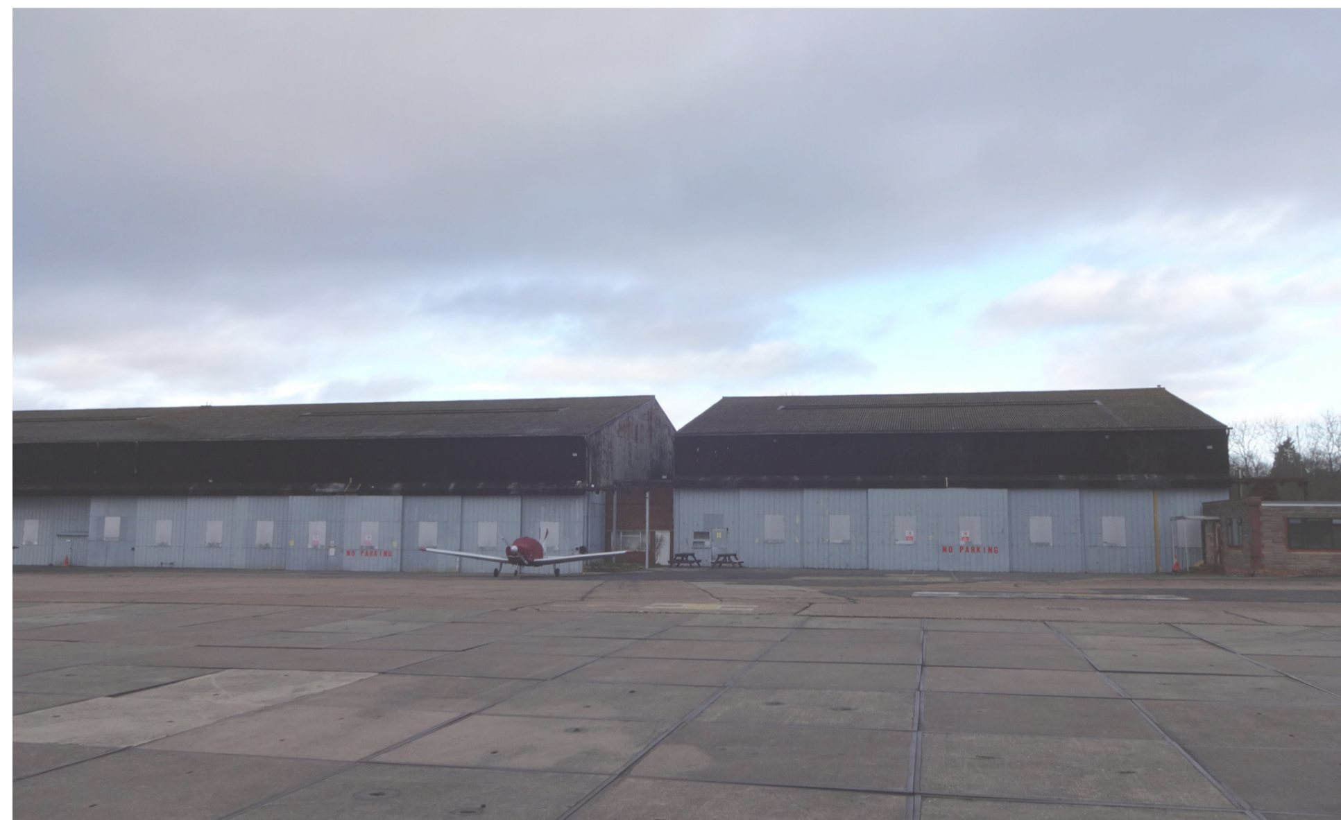
Existing apron and hangars.
