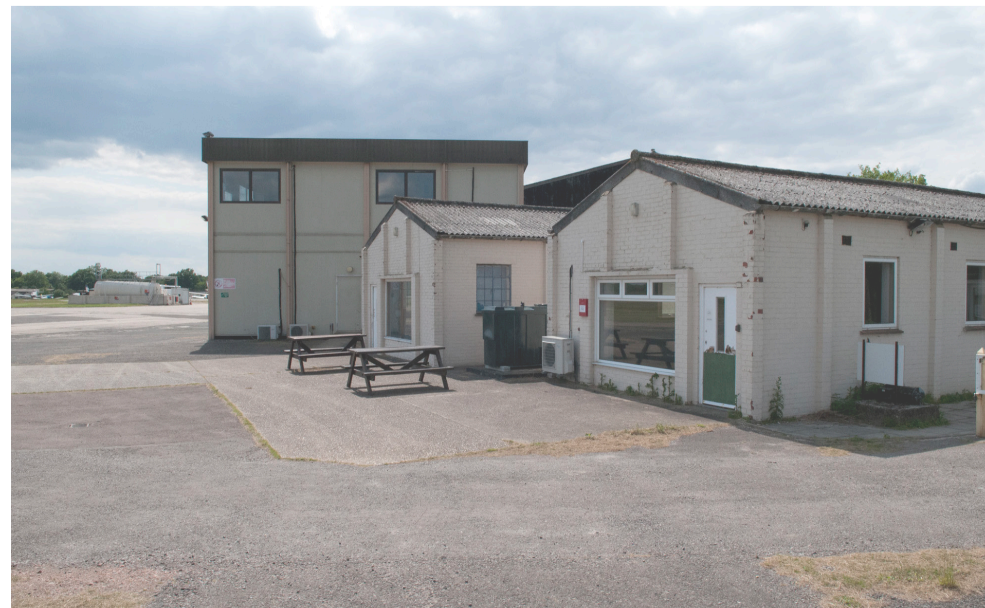
Vacant single and two storey buildings.
