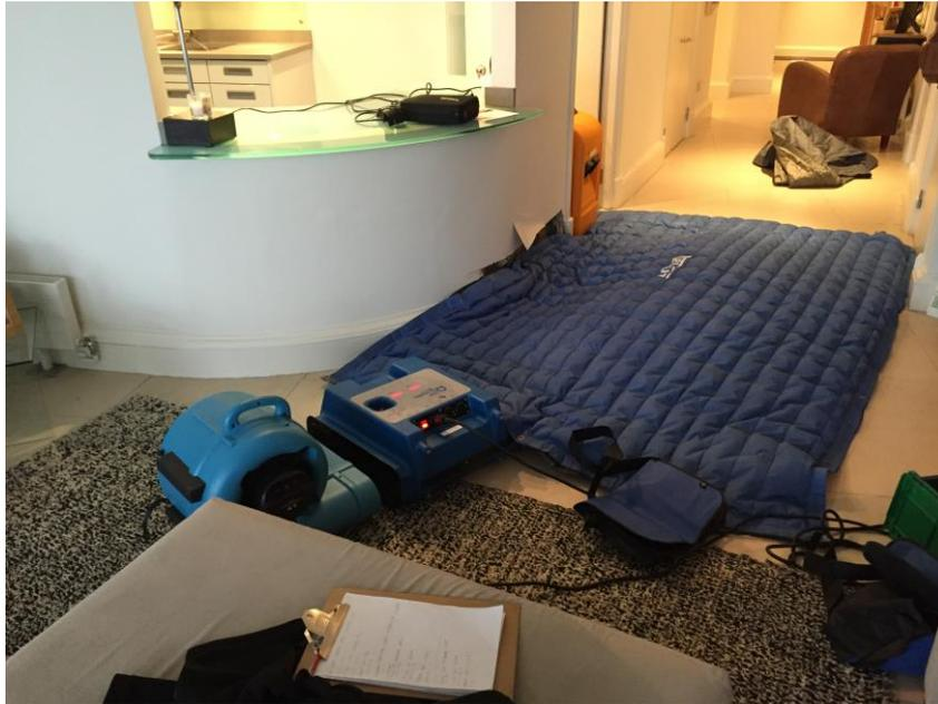
The floor was heated to 34c using a controlled heating process for a period of 15 days and then left to stabilise for a further 5 days.
