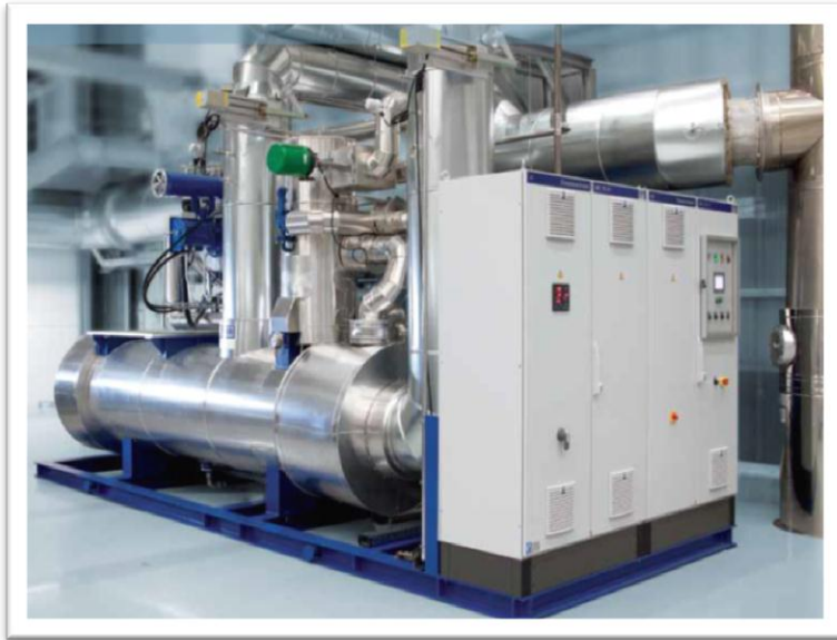
GENERATION: Organic Rankin Cycle Turbines recovery heat from Flue Gas
