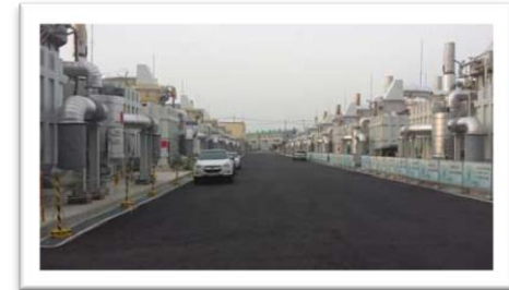
59 MW Gyeonggi Green Energy facility Hwasung City, South Korea.
