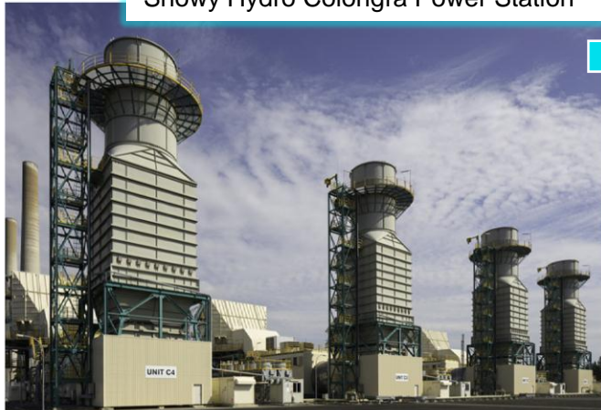
Snowy Hydro Colongra Power Station
