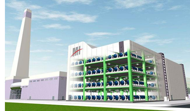
Concept for a large Power Plant based upon Solid Oxide Fuel Cells (SOFC)
