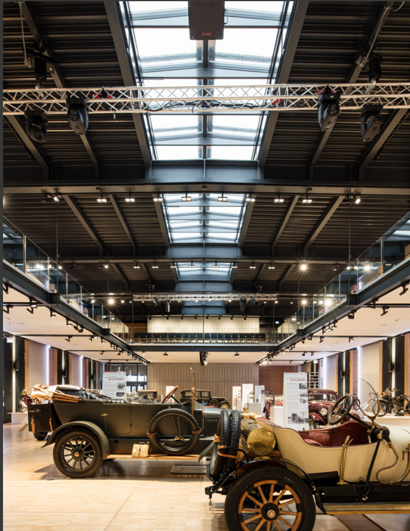
PS.Speicher, Museum, Einbeck, Germany. Ridgelight at 5° with Beams, 50 modules.
