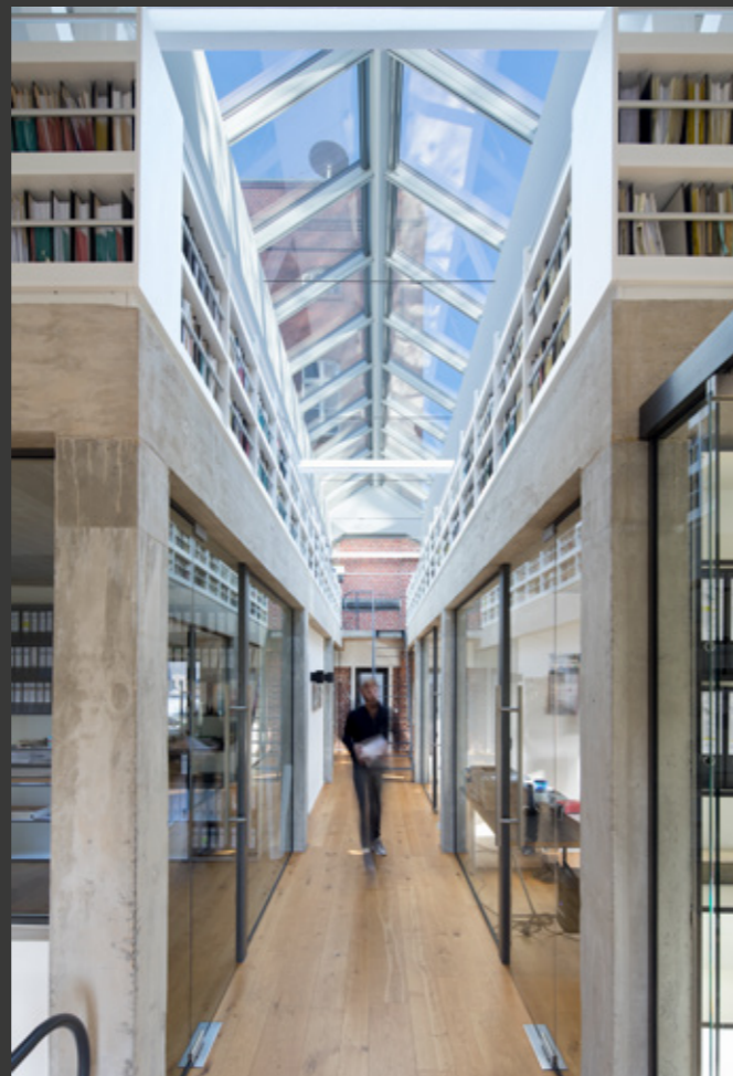
Old Firestation, Architect office, Leverkusen, Germany. One Ridgelight, 22 modules.
