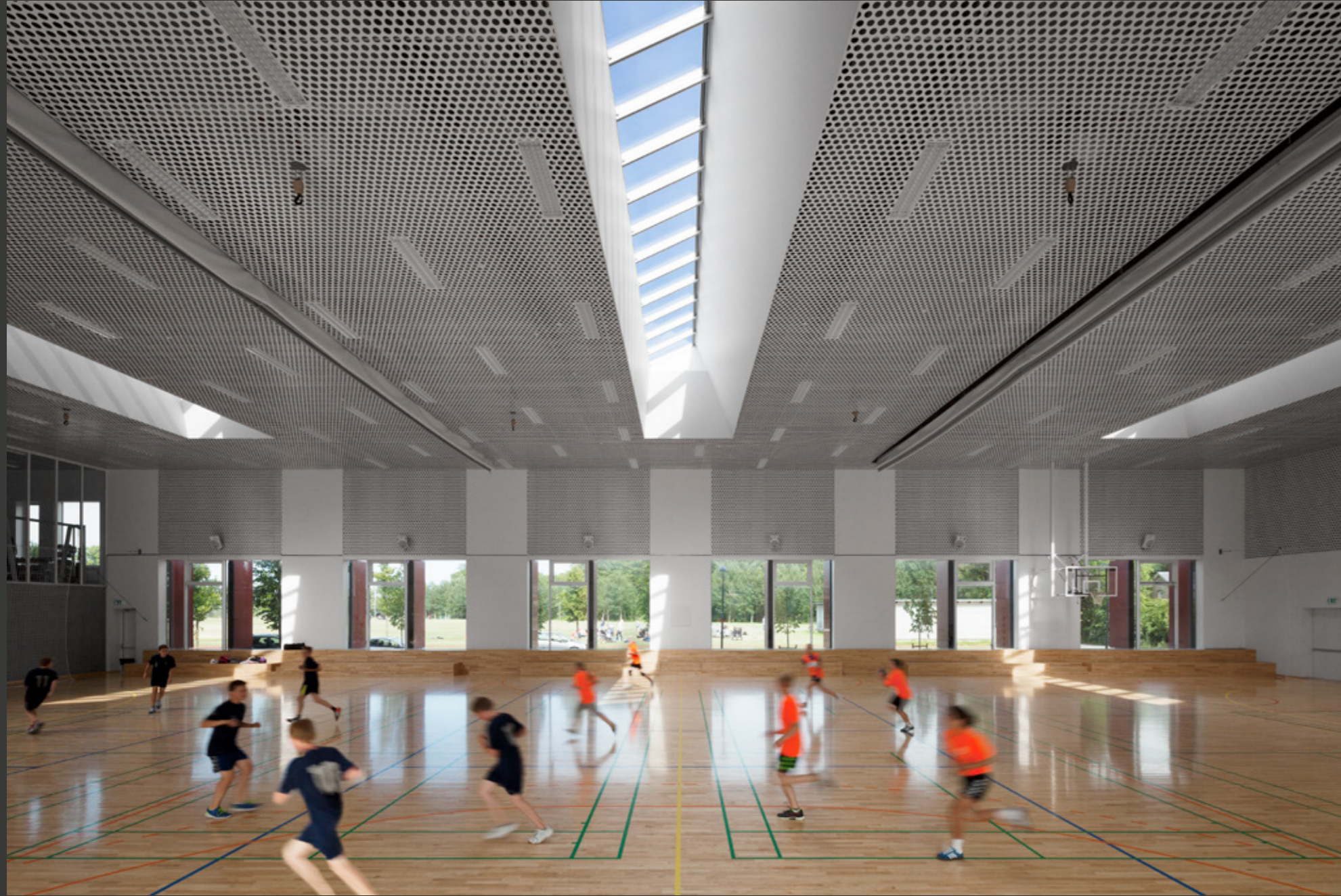
Hal C, Multi Sports Arena, Copenhagen, Denmark. Three Longlights, 60 modules.
