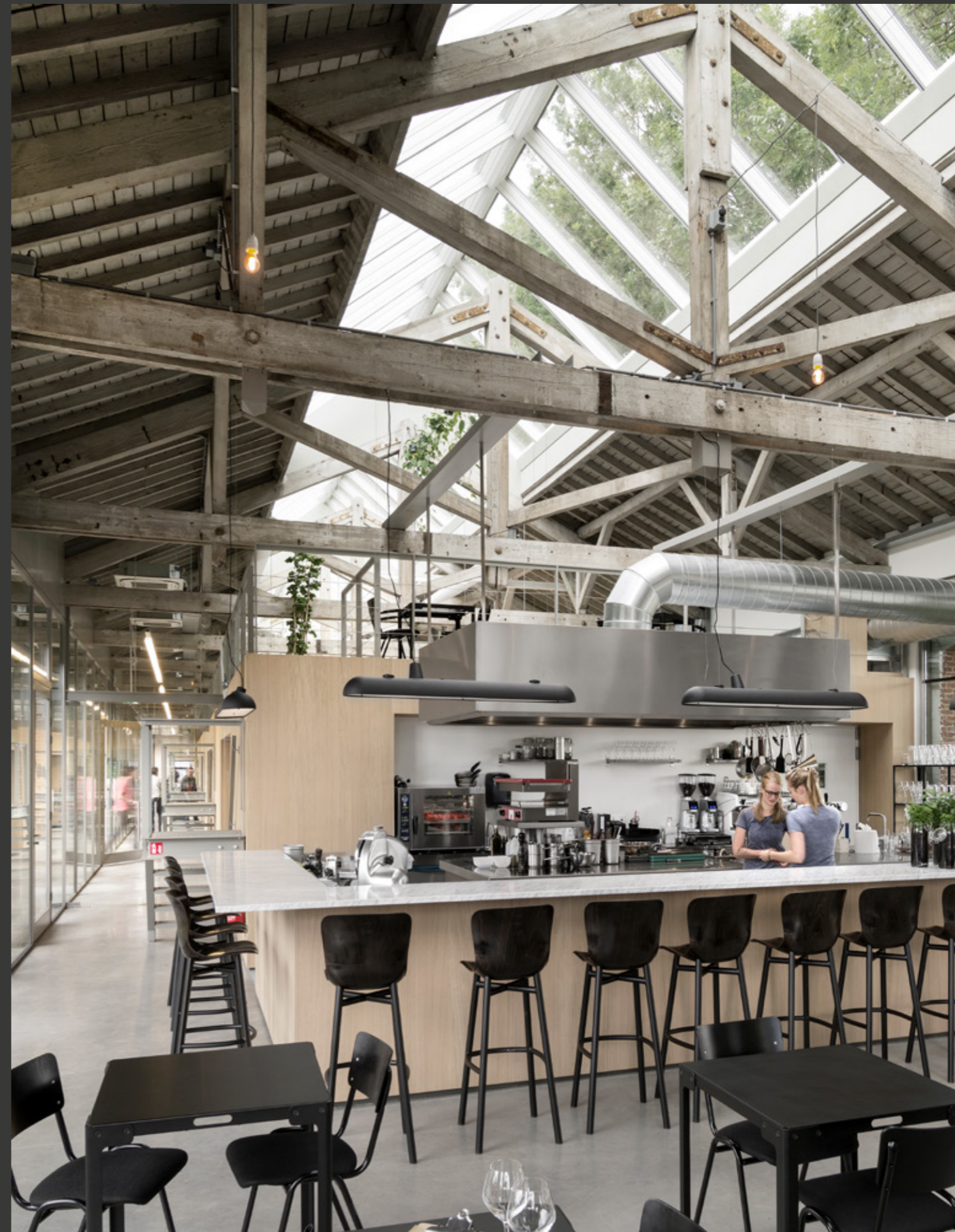
The Houtloods (transformation of old railway warehouse), Tilburg, The Netherlands. One Ridgelight, 124 modules.
