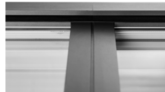
Assembly of middle and top section cladding. Longlight 5-30°.
