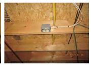
There is a connection for the basement central vacuum that has not been completed
