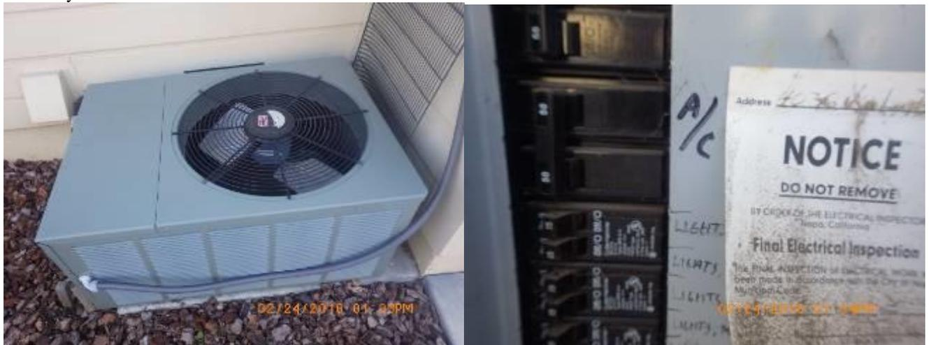
The breaker for the AC unit is oversized for the unit; max 35 amp breaker; 50amp breaker.
