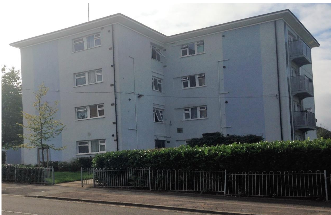
Refurbished flats on Robin Hood Avenue
