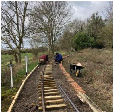
We are now bending rail in situe for the first corner following the main straight. The first three 'outer' rails have been bent and are being connected with fishplates by Tony and Greg.
