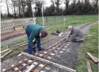
Wednesday 26 Feb saw the final crossover point installed by Mike Williams and his helpers. The photo shows the point connected into the platform 2 track and final levelling taking place.
