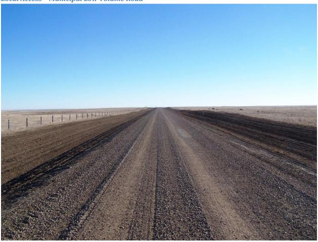
The Municipal Low Volume Road sub-classification is a roadway within an existing government road allowance, whether it be for new construction or re-construction of an existing road to current standards. The minimum basic ROW for this road designation is 20.12m. The Municipal Low Volume Road provides local access to three (3) or less residences or does not permit through traffic.
