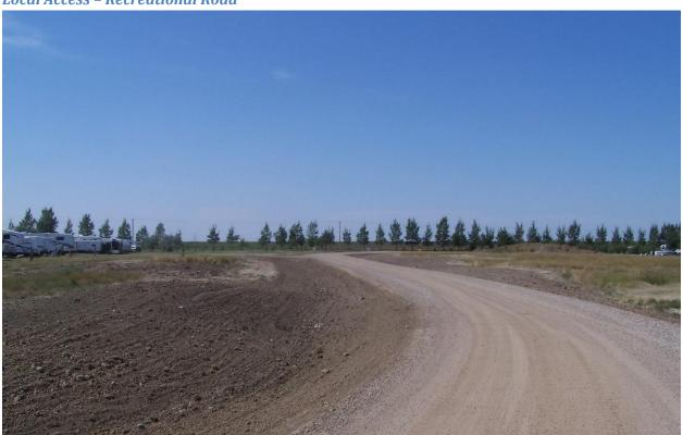
The Recreational Road provides access to land in rural park settings. This type of road may incorporate stormwater drainage, water and wastewater infrastructure and/or other utilities within its cross section as required.
