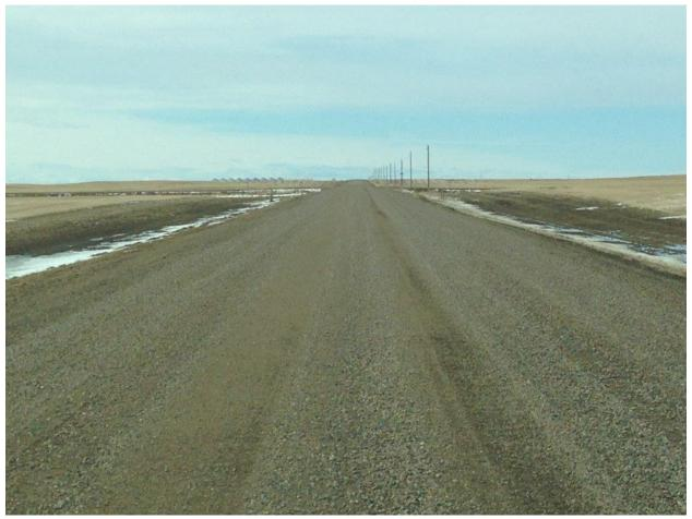
Collectors provide access to land and provide a higher level of traffic movement than Access Roads. Collector roadways collect traffic from Access Roads and channel it to higher classified roadways. The Collector classification applies for roadways with moderate volumes of daily traffic composed of light, medium and heavy-duty trucks and passenger cars.
