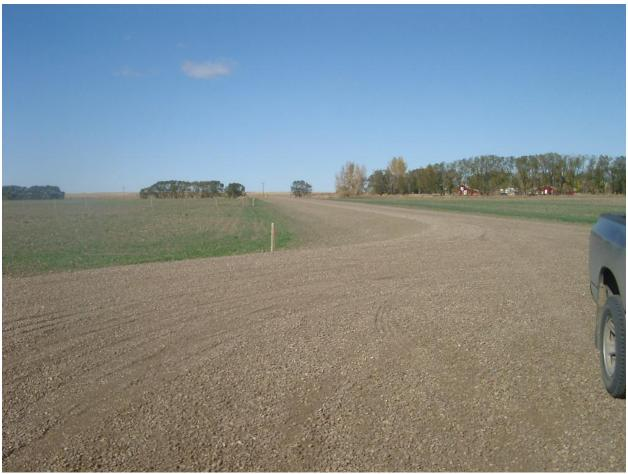
The Internal Subdivision Road provides access to country residential parcels. The basic design for an Internal Subdivision Road provides an oiled 7.6m road surface with 4:1 side slopes and 3m ditches within a 30m right-of-way.
