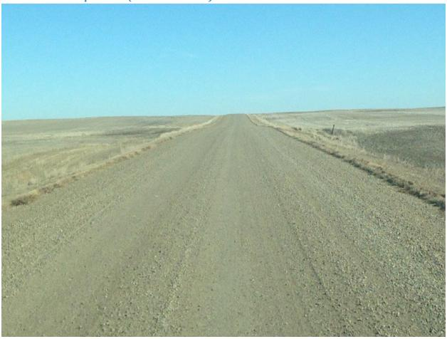
The Municipal Road (Gravel Standard) sub-classification is a roadway within an existing government road allowance, whether it be for new construction or re-construction of an existing road to current standards. The minimum basic ROW for this road designation is 20.12m or 30.18m.
