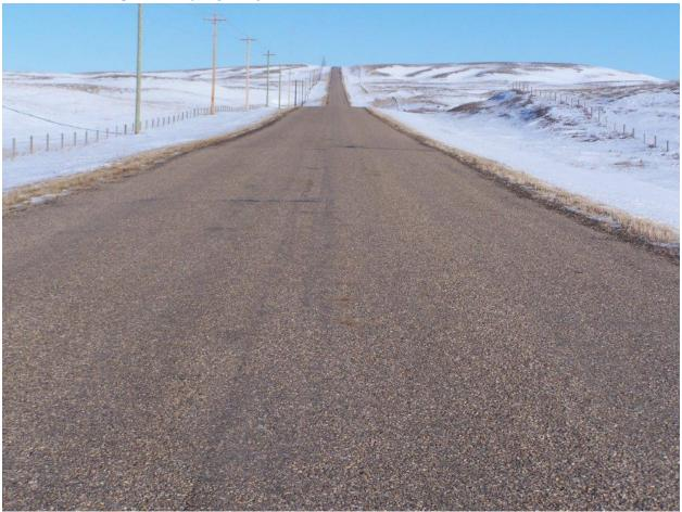
The Municipal Road (Surfaced) sub-classification is a bituminous or concrete roadway within an existing government road allowance, whether it be for new construction or re-construction of an existing road to current standards. The minimum basic ROW for this road designation is 20.12m and preferred ROW is 30.18m.
