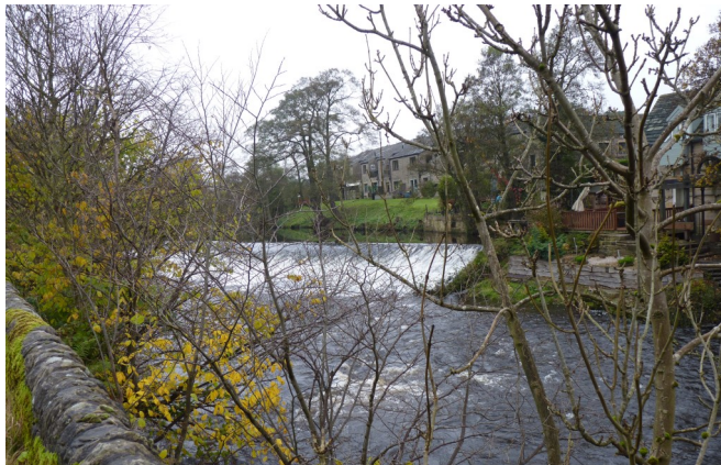
Baslow Weir, Before
