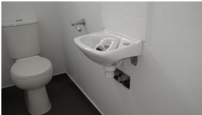
Wall tiles Ceramic Silicon installed instead of grout to top of tiles, should be removed and matching grout installed Condition: Defect Noted
