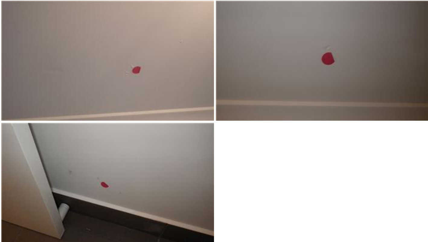
Walls Plaster Marks noted to walls where indicated that require removal or painting Paint runs noted that require sanding and touch ups Condition: Defect Noted
