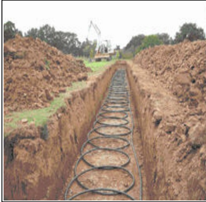
Slinky coils laid horizontally in trench
