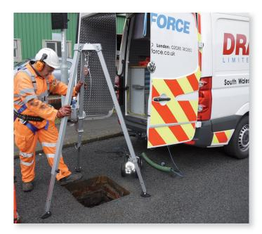
Drainforce currently operates two fully equipped survey rigs, capable of surveying manholes in both rural and major traffic areas. All of our Manhole surveyors are trained to WTI standards and are capable of producing high quality reports in current STC25 format.
