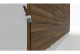
Because the cut ends of boards tend to draw moisture into the wood more quickly than the other surfaces, it is highly recommended that more than one coat of wood preservative be applied to these.
