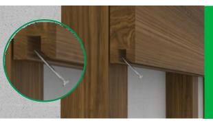
For tongue and groove cladding installation, it is recommended to use an air gun to drive in stainless steel nails.
