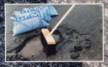
PREPARE the area by sweeping and removing loose debris.
