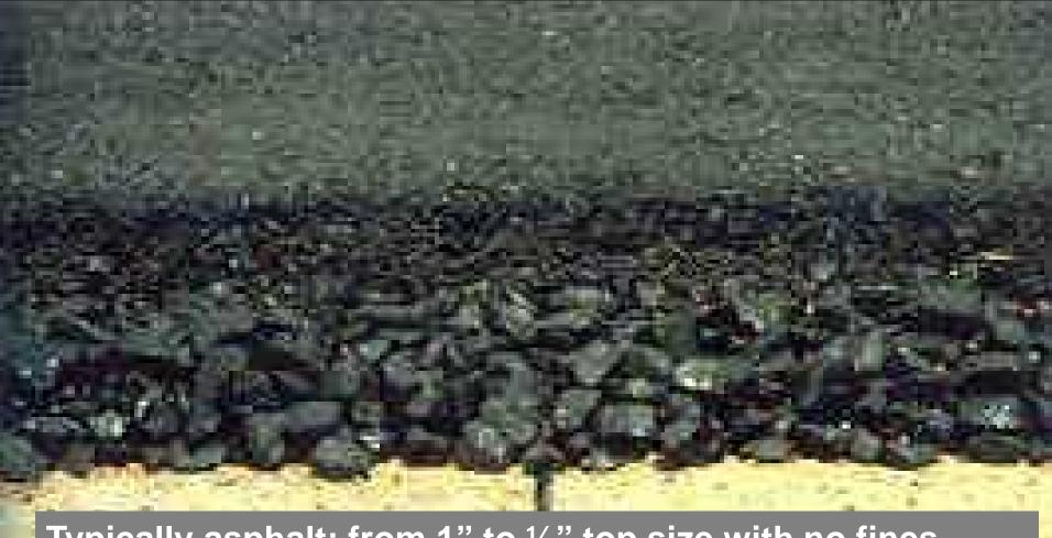
Typically asphalt; from 1" to  $\frac{1}{2}$ " top size with no fines. May be aggregate base.
