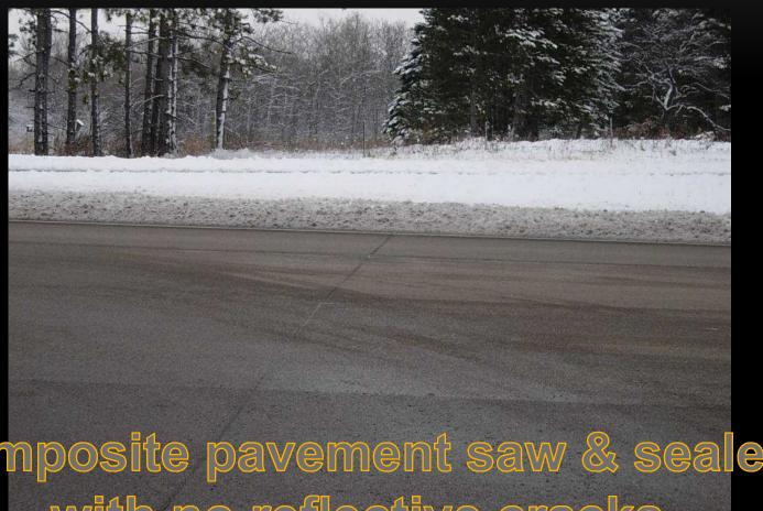
Composite pavement saw & sealed with no reflective cracks
