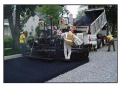
The intersections were constructed in September 2010. Midwest Asphalt Corporation was the paving contractor (see photo above). One complete winter of monitoring and observation has occurred (see photo of snow melted on porous asphalt pavement section to the right) and the results look promising for the use of porous asphalt as a physical means to reduce salt. What we've seen is
