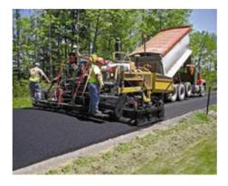
In addition, WMA technologies allow asphalt mixtures to be hauled longer distances and can extend the paving season due to WMA's ability to maintain workability at lower temperatures. The proper use of WMA may result in reduced overall paving costs.
