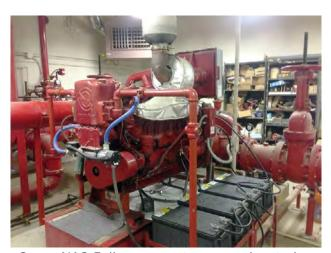
Some NAS Fallon generators were located deep in building basements to power fire control systems or as auxiliary power backup systems. Installation of FloScan systems on these generators was extremely simple.
