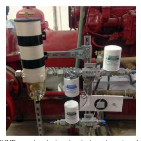
JHME constructed a simple tree-type bracket for the FloScan supply and return line sensors and Fuel Log gauge then attached the fuel lines to complete the installation.
